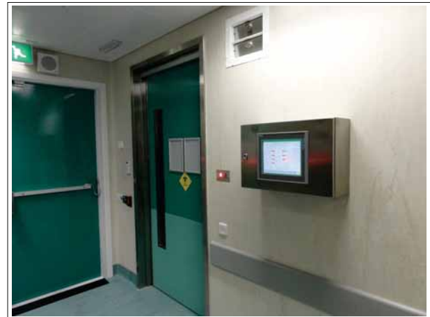
LED-225 alarm indicator plate with buzzer on wall
