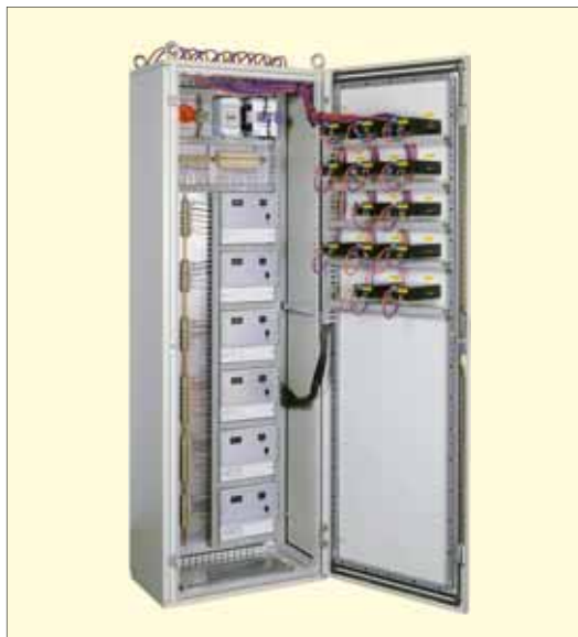
Internal view of the CMR Panel. An isolator, fuses, power supply, computer interface terminals and six DPC100 Controllers are fitted on the back plate. All factory tested.
