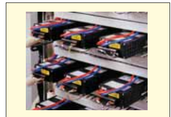
CMR panel door showing the rear of the DPMs. Designed for easy access during calibration in future.
