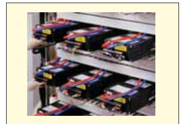
CMR panel door showing the rear of the DPMs. Designed for easy access during calibration in future.
